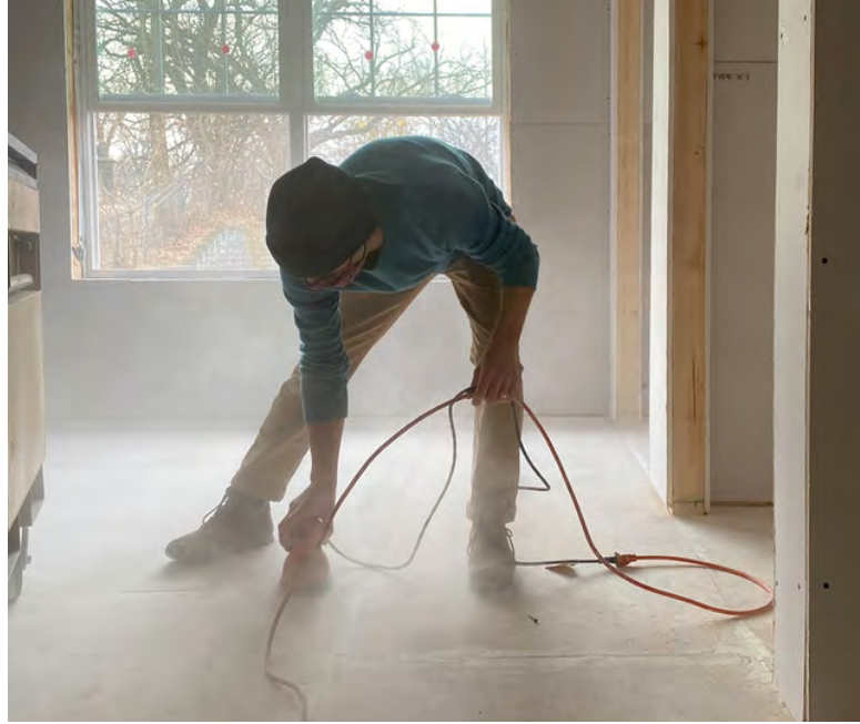
Sanding floors in preparation for tiling.
