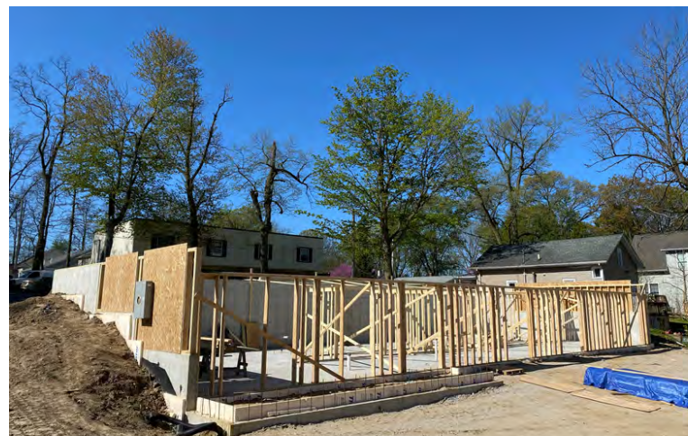
Respite House II - first floor framing.
